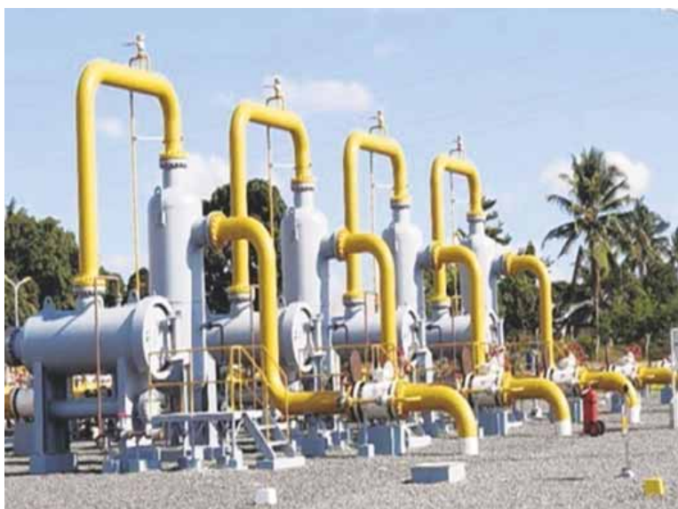
Photo: Gas Pipeline Project, Mtwara, Dar es Salaam
